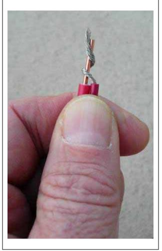
3 - Twist the wire nut onto the wires until it is very tight.
